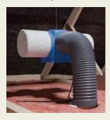
This is a simple option but can have high running costs (electricity) and may cause comfort issues when cold air is forced into rooms. There is an additional structural risk in forcing warm and moist air into the building fabric.
